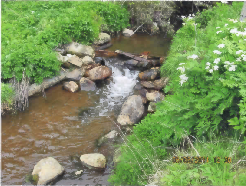
Pic 1 Small weir dismantled, Before
